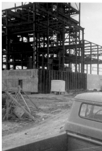
Holly construction, circa 1960
